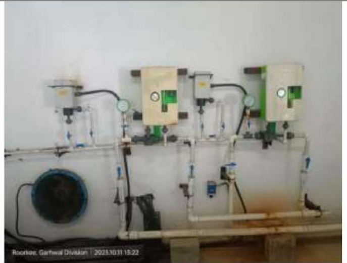
Fig 6: Gas chlorinator
