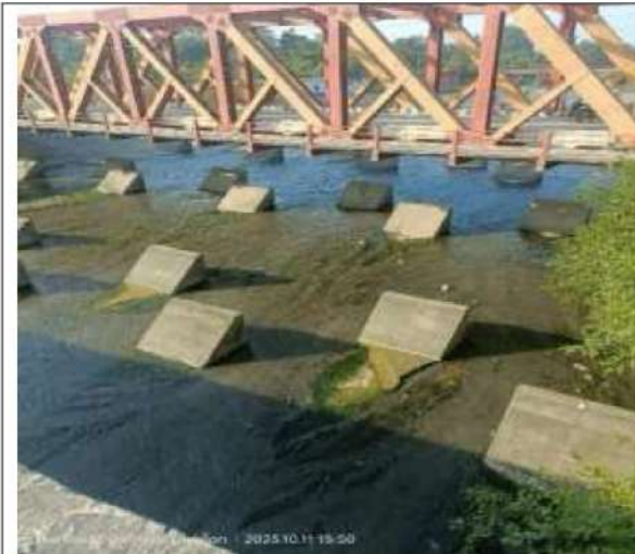
Figure 18: Sukhi or Roe River at Bridge on National Highway Bahadarabad
