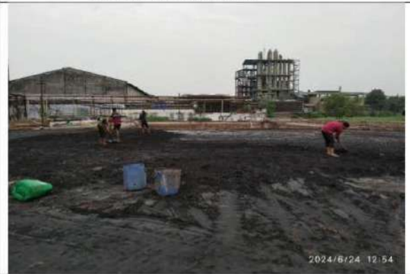
Photo 10: Lagoons filled/levelled with ash and covered with brick lining
