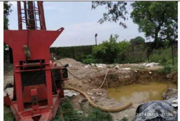
Photo 9: New borewell for distillery plant under installation
