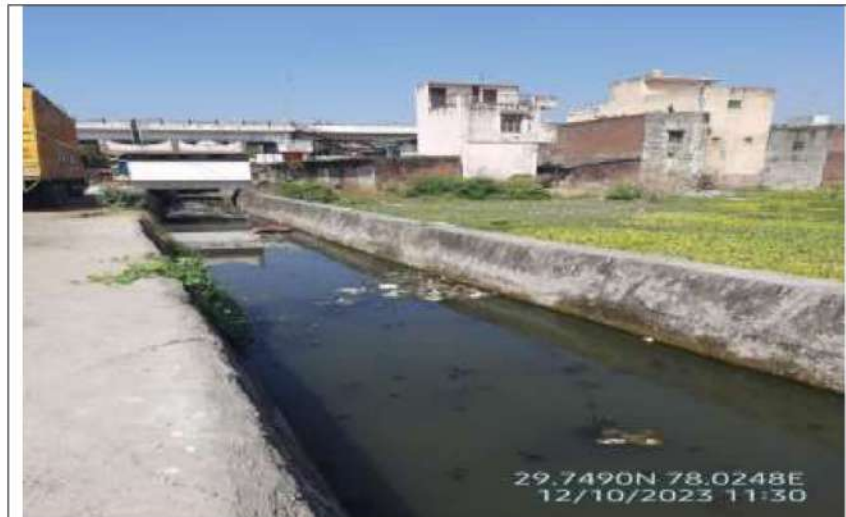
Figure 27: Laksar drain near railway track (upstream of unit)
