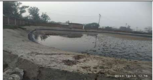
Photo 16: Spent wash storage in bio-compost yard
