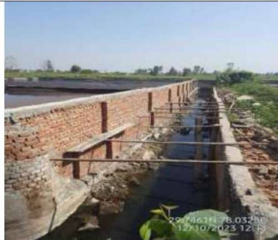
Figure 30: Laksar drain near lagoons of the unit
