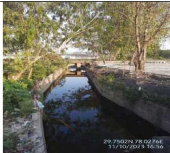
Figure 28: Laksar drain upstream of unit
