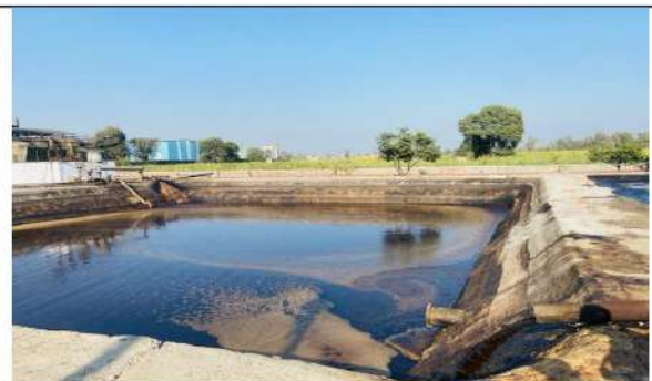
Photo 20: Lagoon for storage of conc. spent wash
