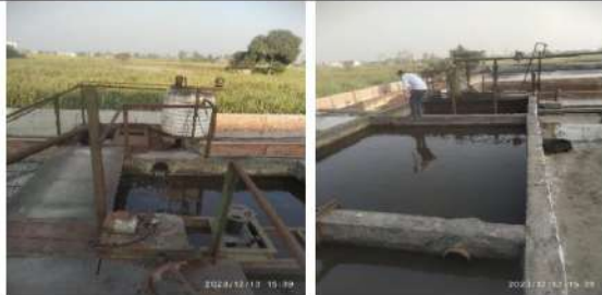
Photo 13: Alum dosing and tube settler
